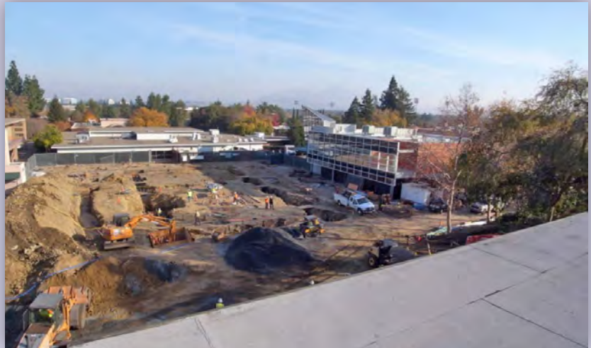
Here is the photo captured on December 6, 2011, by one of two webcams pointed at the DVC Commons Project construction project.
